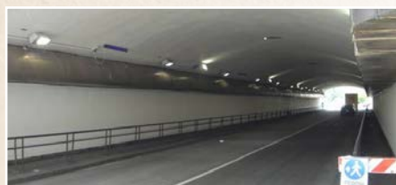
An extreme test: Urban tunnel in Milan. (Via Porpora) State of the Photocatalytic wall (left) and untreated area (right), after a month of traffic.
