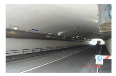
Tunnel with blue UV fluorescent tubes to activate the cleaning effect
